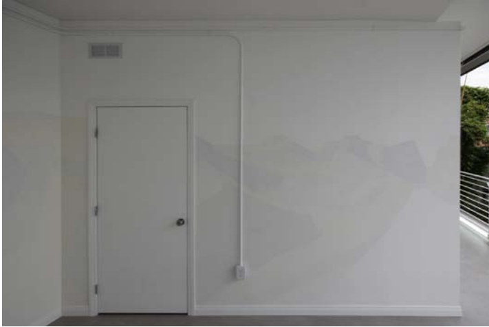
New wall with mountain panorama, molding, and conduit.
